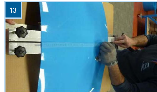
13 Clean the weld on this side too.
