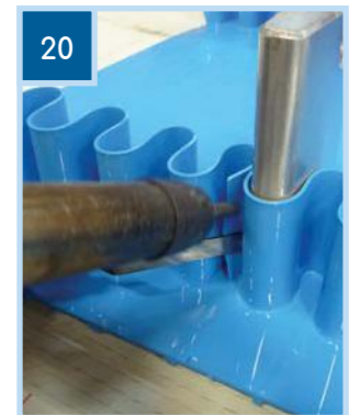
Re-Welding the Sidewalls Re-Weld the Sidewall to the belt using a hot air gun (Figure 19 & 20).
