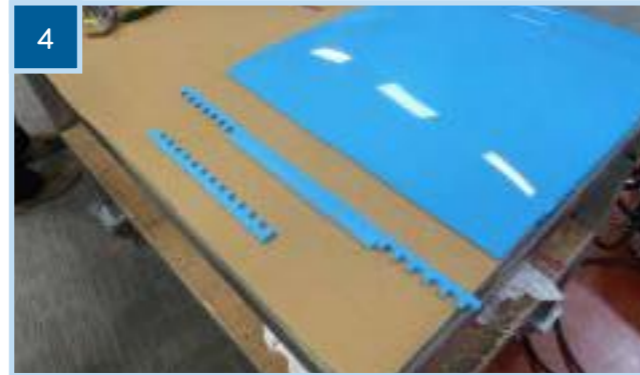
4 As can be seen, a single module has been placed opposite the measured lace edge. The remaining sections on either side of this module should now be cut to size.
